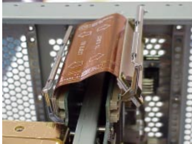
Figure 4-50. The Flex Cable Disconnected from the I/O Board Side
